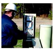
FIBRBox splice enclosures offer TE Connectivity's proven fiber splice management and organizing performance in a rugged enclosure designed for today's FTTx applications. FIBRBox splice enclosures combine a corrosion-resistant enclosure, gasket and grommet entry points, and the familiar stair-stepped, hinging tray design in an enclosure that will accommodate two feeder cables and up to sixteen drop cables (depending upon the drop cable design).
