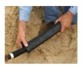
2 Cable End Seal & Jacket Repair
