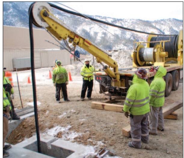
970' vertical single-messenger MPF borehole installation.
