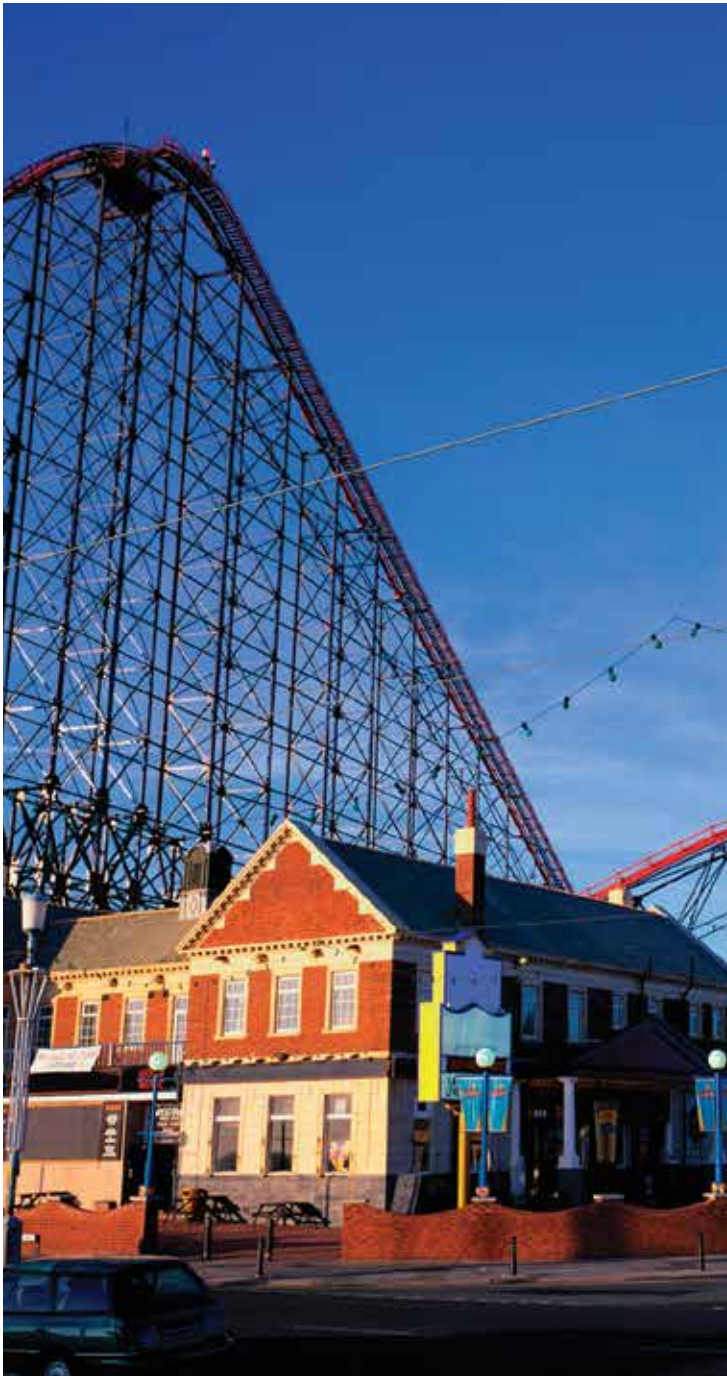
DR Horns Can Be Deployed In Amusement Parks As Part Of A High Intelligibility Paging System
