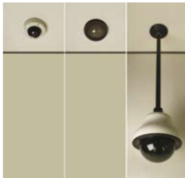
Figure 4.6a An example of a surface mount (left), a flush mount (middle) and a pendant mount (right).
