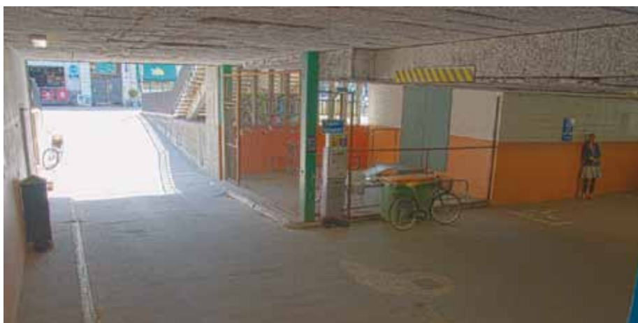
Figure 9: Parking garage, indoor. The image is taken from an Axis camera that incorporates the WDR-dynamic capture technology.
