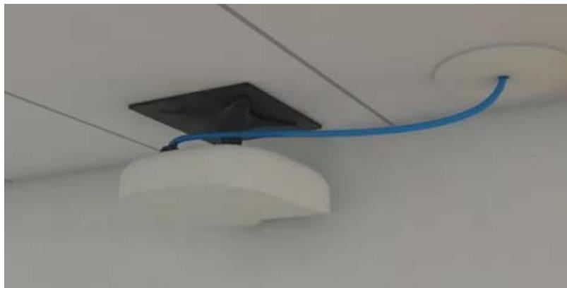
**Figure 2 - Direct Connection Outside Plenum Space**
