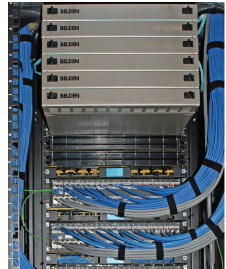
Belden’s ability to customize solutions to meet the needs of the hospital verified that MaineGeneral selected the right partner. For example, after the hospital realized that some servers required Category 6A to support 10 gigabit Ethernet, Belden was able to accommodate six 10GX Category 6A ports (gray) alongside the existing Category 6 (blue) in patch panels within the server distribution area.
