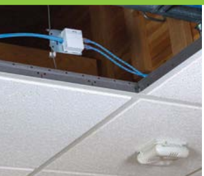
Plenum-Rated QuickPort™ In-Ceiling System
