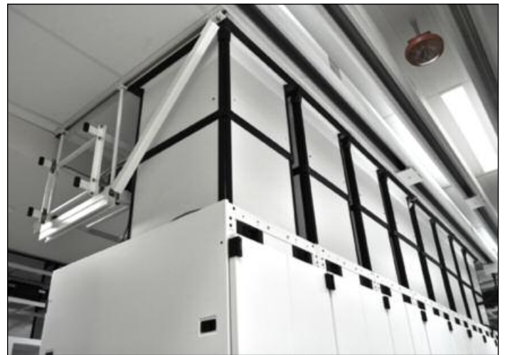
Vertical Exhaust Ducts direct heated return air into the plenum space, which isolates hot and cold air to create a containment solution that increases efficiency of both KyotoCooling® and traditional cooling systems.
