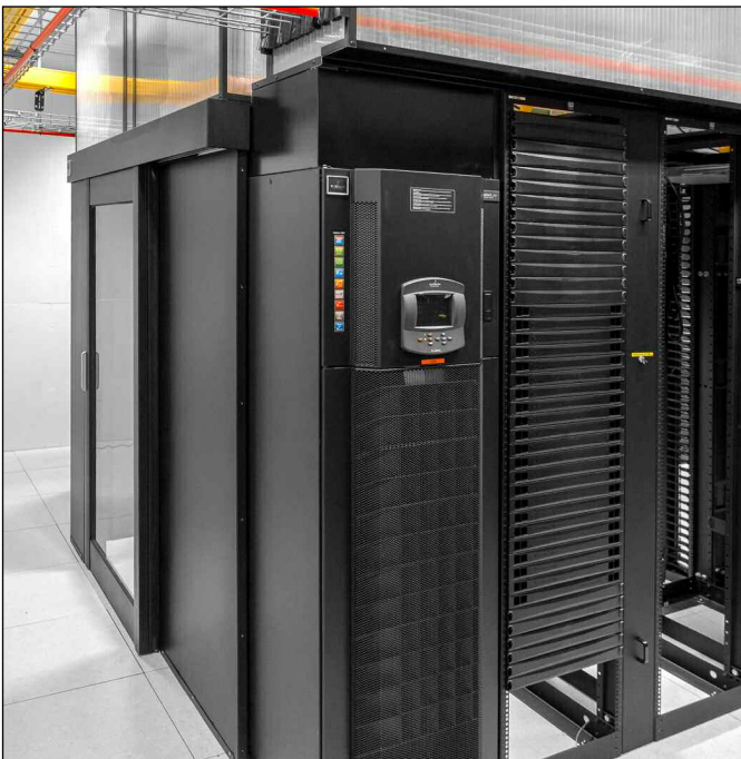
Evolution® Cable Management, Four-Post QuadraRacks, Aisle Containment Door Systems and Brushed Grommets were used to build a flexible solution that could be assembled on site.
