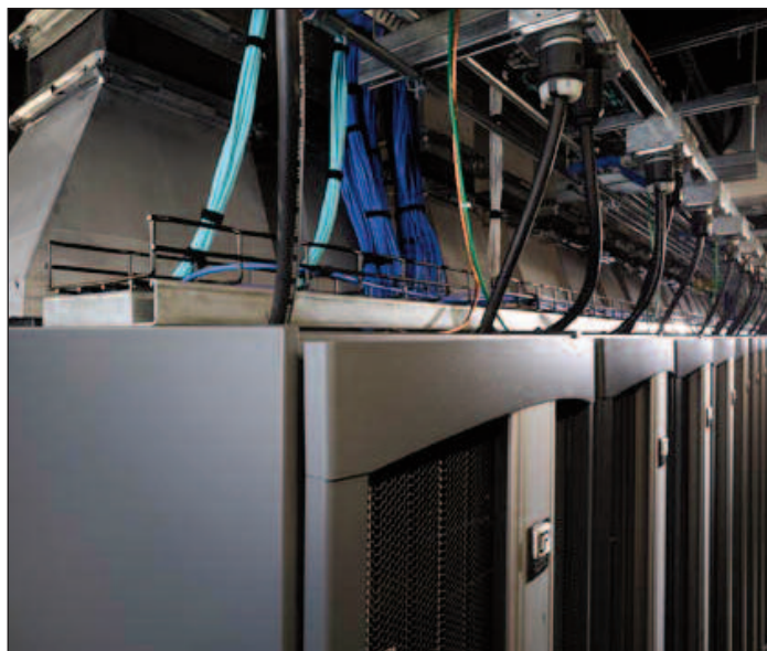
CDW has installed 103 F-Series TeraFrame Cabinets with Vertical Exhaust Ducts in the first phase of their new data center.
