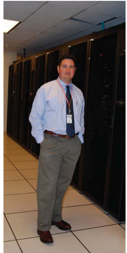
Russell Lowery, Senior Network Engineer, Telecommunications for GHS in data center
