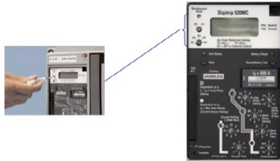
Figure 6 Air circuit breaker included an integral trip unit with Arcflash Reduction Maintenance System (ARMS) capabilities.
