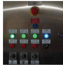
Figure 9 The SCADA system includes reset access to DOL motor loads so that operators can reset thermal overloads remotely (left image). Circuit breaker controls and ARMS activation is from the remote panel mounted in the airlock room adjacent to the main switchroom.
