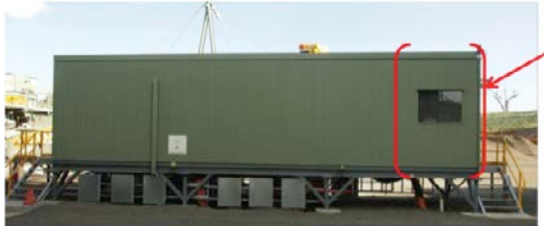
Figure 8 The main switchroom is designed with an airlock section where the ARMS switch and confirming indicating light are mounted. This functionality is activated prior to maintenance persons gaining access to the main switchboard area.
