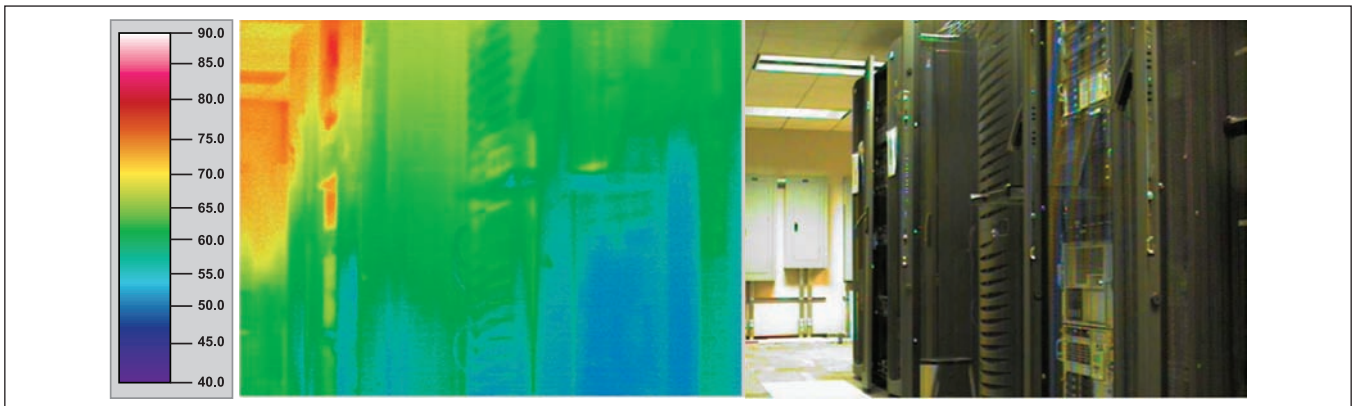
Figure 1: Thermal Imaging of Rack Inlets
