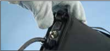
Fig. 26 Using the ERICO CADWELD EXOLON battery pack, press the button. At this time, the unit will send a charge to the igniter pin. The igniter pin will initiate the ERICO CADWELD EXOLON exothermic reaction.
