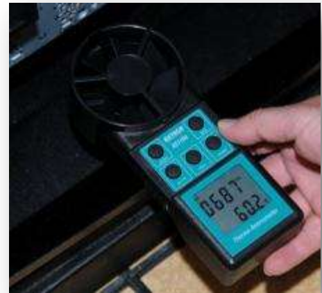
Anemometer showing feet per minute and air temp in Fahrenheit
