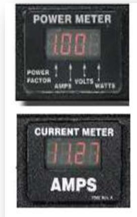
Metered PDU readouts help balance phases and calculate power usage
