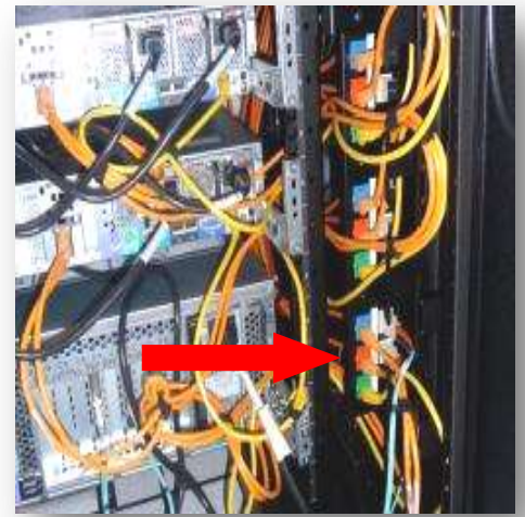
Zero RMU mounting of patch using Vertical Patch Panel
