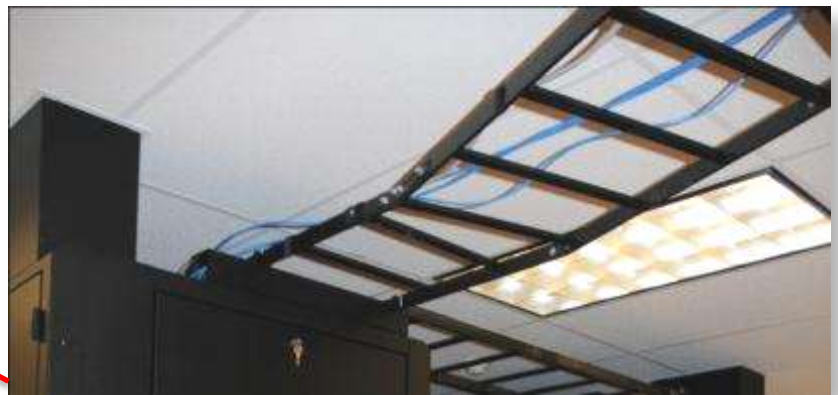
Ladder Rack Brackets support the overhead cabling system saving the need for overhead suspension systems and removes hanging stanchions making accessing cables easier
