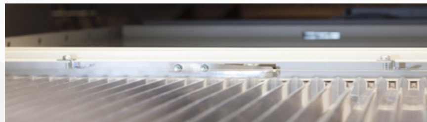
Bonding of drop away panels
