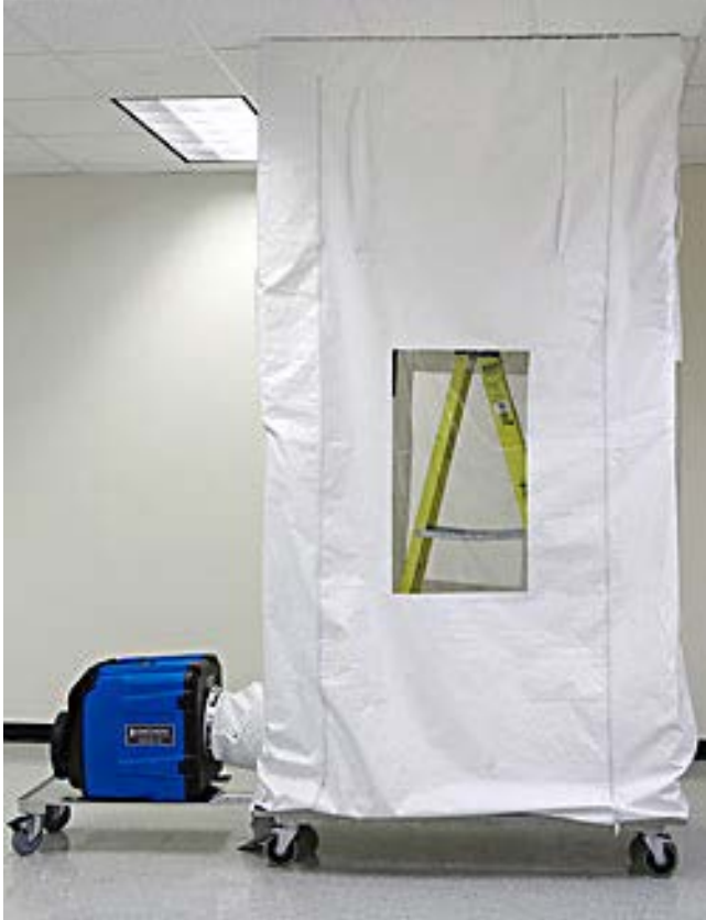
When ceiling tiles are lifted, and work is being performed, the work area shall be tented and negatively pressurized.
