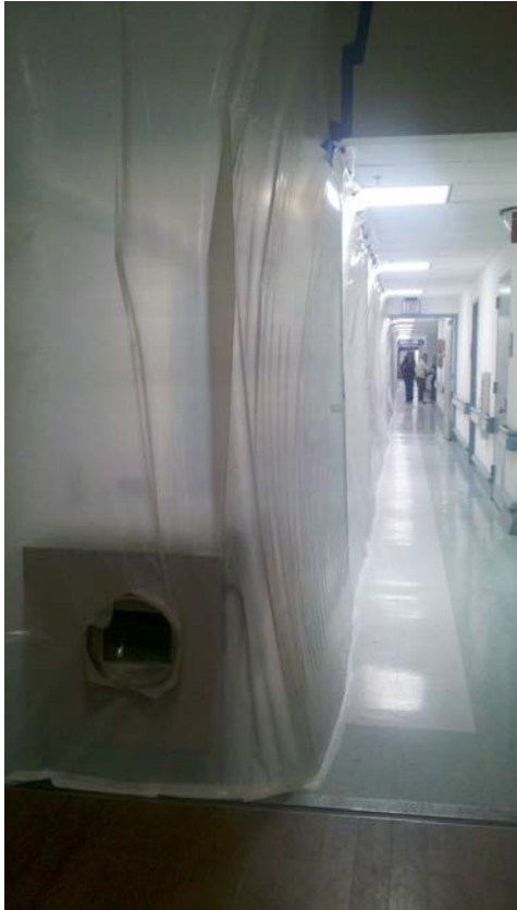
When ceiling tiles are lifted, and work is being performed, the work area shall be tented and negatively pressurized.
