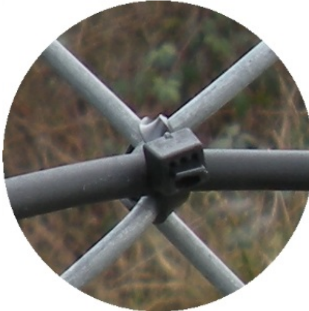
Figure 4-2. Correctly tied through vertically adjacent diamonds.
