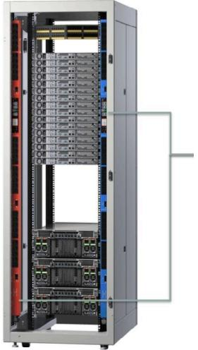
RCM Technology included inside the intelligent PDU at the rack level
