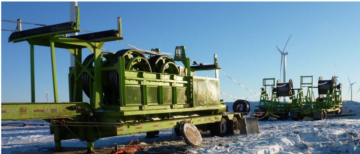
Figure 6. Payoff and bullwheel setup.
