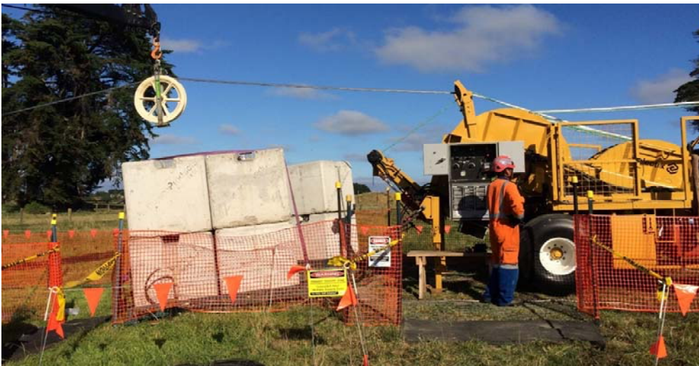
Figure 10. Suitable technique for roller diversion, courtesy of Transpower New Zealand.
