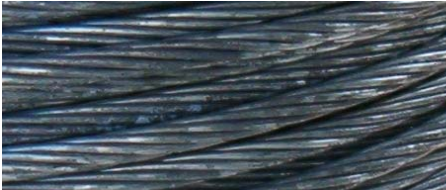
Figure 4. Oxidation on a conductor.
