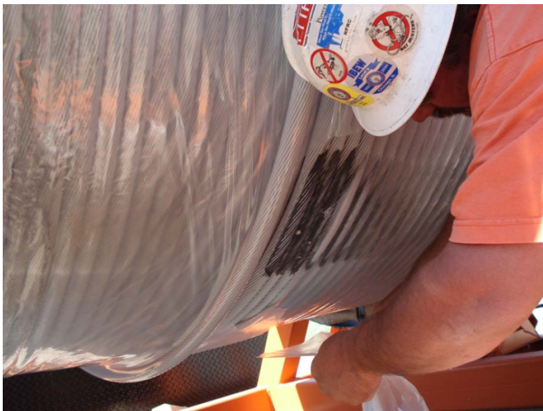
Figure 5. Water stain on conductor.
