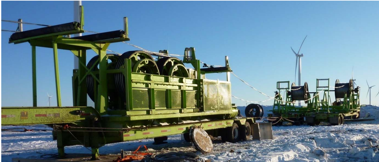
Figure 5. Payoff and bullwheel setup.
