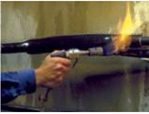
Polymeric wye and H-tap splices produce dependable water tight seals between the main and tap cable(s) with no taping.
