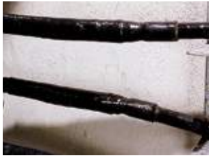
Heat shrink, high-voltage splice kits install quickly and uniformly.
