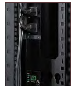
Vertical Rackmount PDU (0U)
