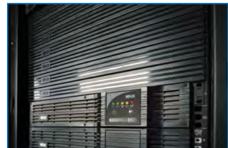
Simple steps like installing blanking panels in unused rack spaces can help prevent warm air from recirculating and improve cooling efficiency.
