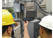
At the RRU (tower structure or rooftop)
