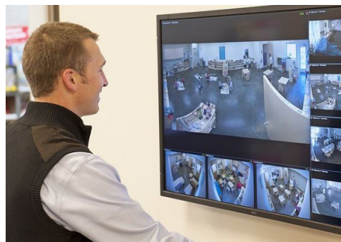
Stone Security testing a newly installed video surveillance system. Photo credit: Stone Security
