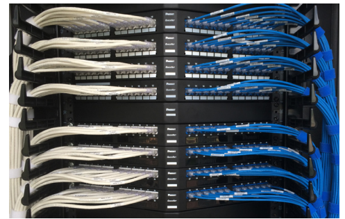
Mini-Com 48-port high-density patch panels are an ideal solution in areas where rack or cabinet space is an issue.
