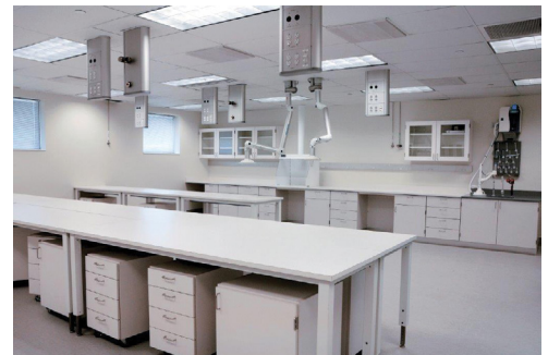
Delivering power, communications and a whole lot more into a healthcare environment.
