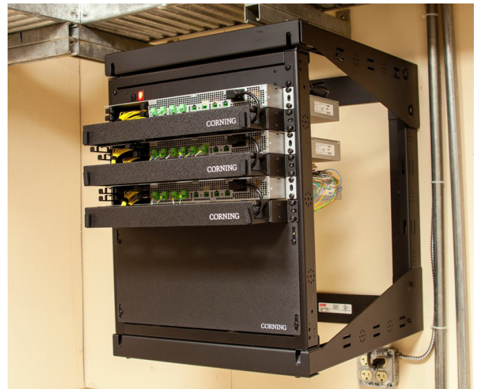
IDF Configuration with Interconnect Unit (ICU)
